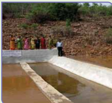
Check Dam at Mandlavanipalli Village, Dhone, Kurnool (ICRISAT)
